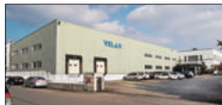
Ansan City, South Korea Velan Ltd., Plant 2
