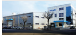
Ansan City, South Korea Velan Ltd., Plant 1
