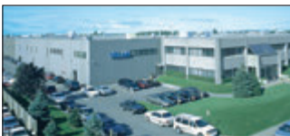
Montreal, Canada Velan Inc., Plant 2 and 7
