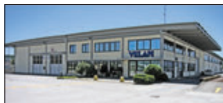
Lucca, Italy Velan ABV S.r.l., Plant 2
