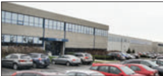
Montreal, Canada Velan Inc., Plant 1
