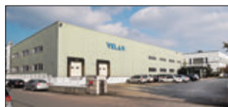
Ansan City, South Korea Velan Ltd., Plant 2
