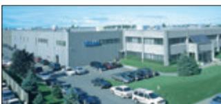
Montreal, Canada Velan Inc., Plant 2 and 7
