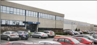
Montreal, Canada Velan Inc., Plant 1
