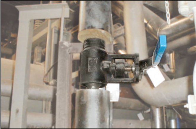
NPS 1½ (DN 40) Power Ball valves in steam trap isolation at a major British power plant. Switching to Velan's Power Ball valves offered a low torque, easy to operate solution.
