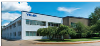
Williston, VT, U.S.A. Velan Valve Corp., Plant 3
