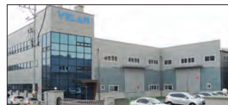
Ansan City, South Korea Velan Ltd., Plant 3
