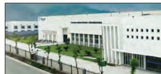
Suzhou, China Velan Valve (Suzhou) Co., Ltd.
