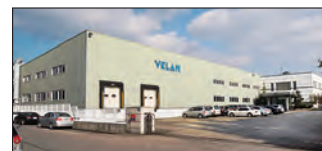
Ansan City, South Korea Velan Ltd., Plant 2
