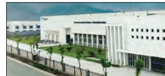
Suzhou, China Velan Valve (Suzhou) Co., Ltd.
