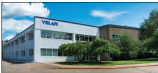
Williston, VT, U.S.A. Velan Valve Corp., Plant 3
