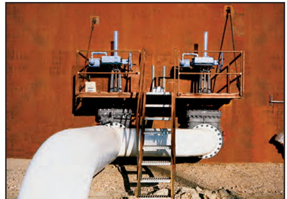
Cast steel valve installation at an oil refinery.
