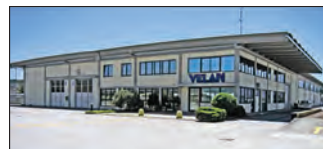
Lucca, Italy Velan ABV S.r.l., Plant 2
