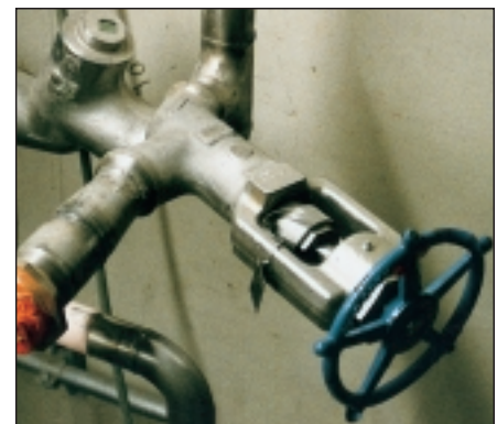
Class 2500 hermetically-sealed Y-pattern bellows sealed valves.
