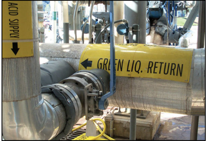
Split-body ball valve in pulp and paper.
