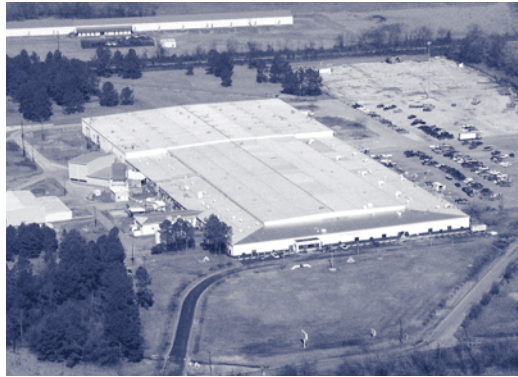
Vogt Valves, Sulphur Springs, TX
